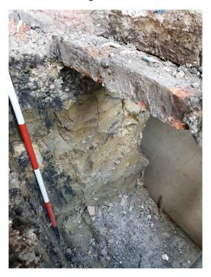
Photo 10. Slag foundation base (red arrow)
